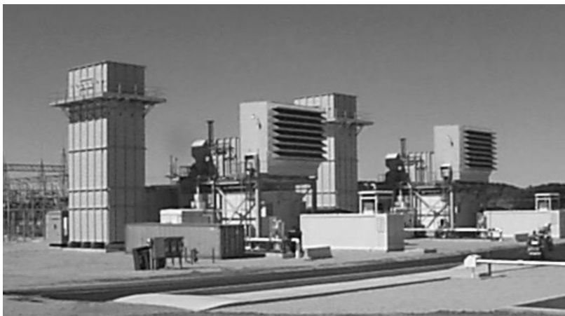
Dairyland’s new Elk Mound gas combustion power plants will help the system provide peak power during high usage times and will also improve Dairyland system reliability.
